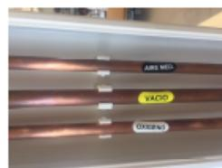
The Gas pippes for medical gases are supplied with certified copper tube and marked according the Gas type
